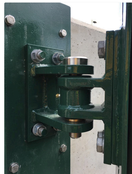
Precision-machined hinge assembly with brass bearings and stainless steel pin, shown installed on a double swing flood gate.
